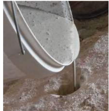
Figure 33 : Coulée de Ciment Expansif
